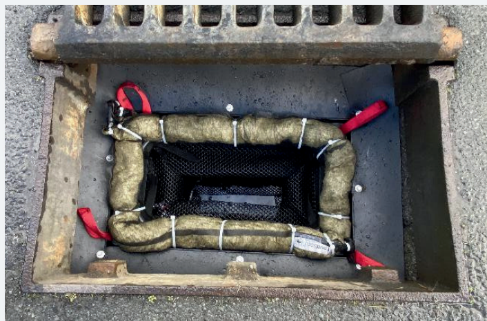
LavaSorb™ Boom set up with EnviroPod™ LittaTrap™ to ensure it absorbs the oils and oil-based liquids.
